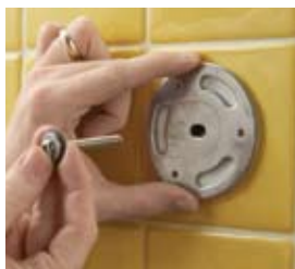
Attach mounting plate to anchor.
