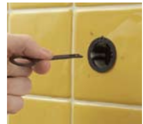
Pull tab until anchor is tight, remove tab.
