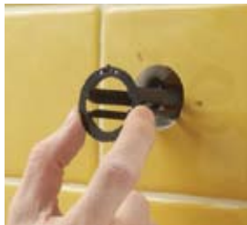
Insert guide sleeve.
