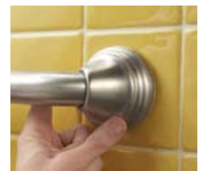
Snap flange cover over flange.
