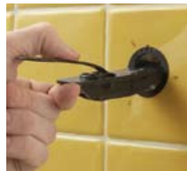
Insert anchor with pull tab into guide sleeve.
